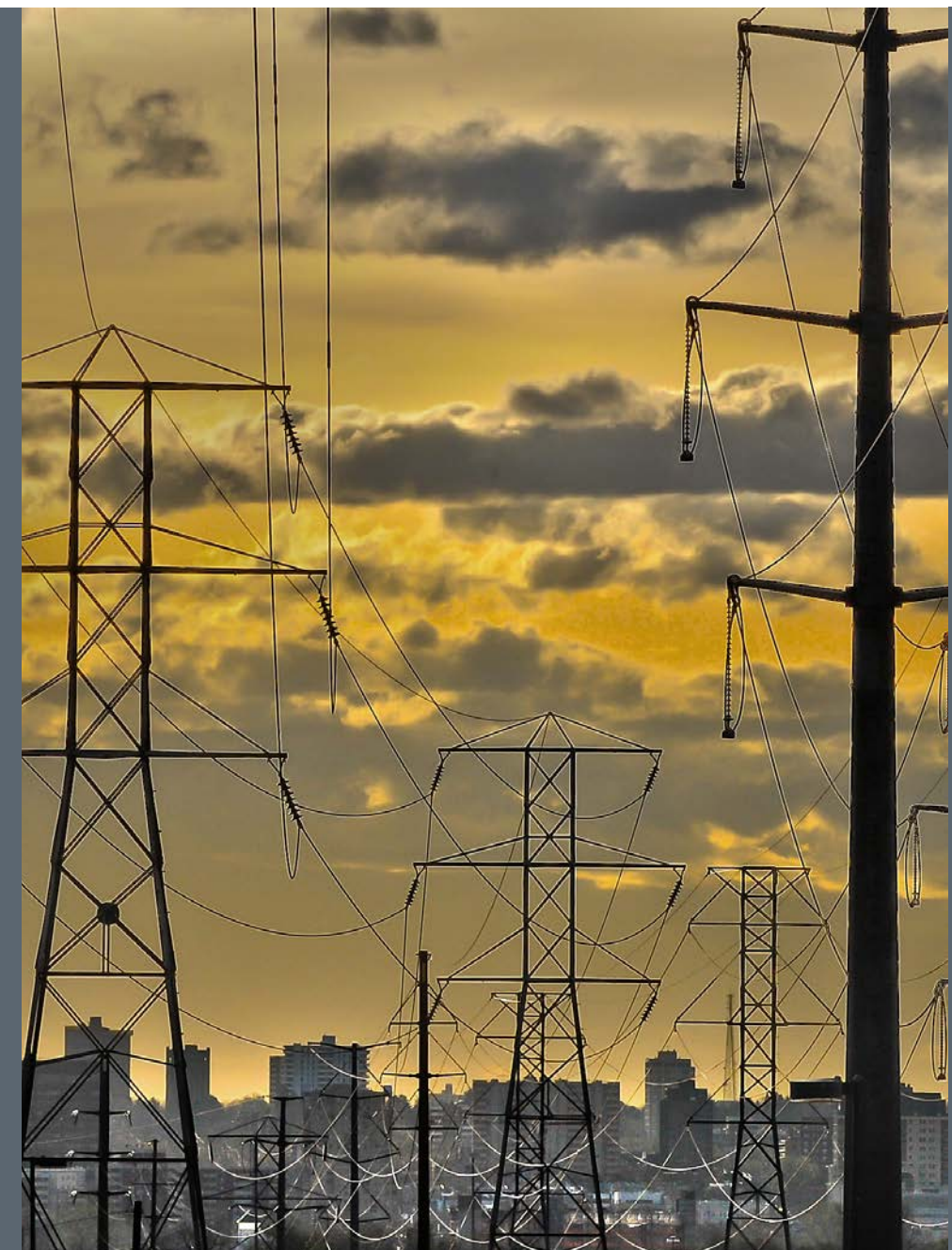
Power lines in Denver, Colorado. Photo by Dennis Schroeder, NREL 18975
