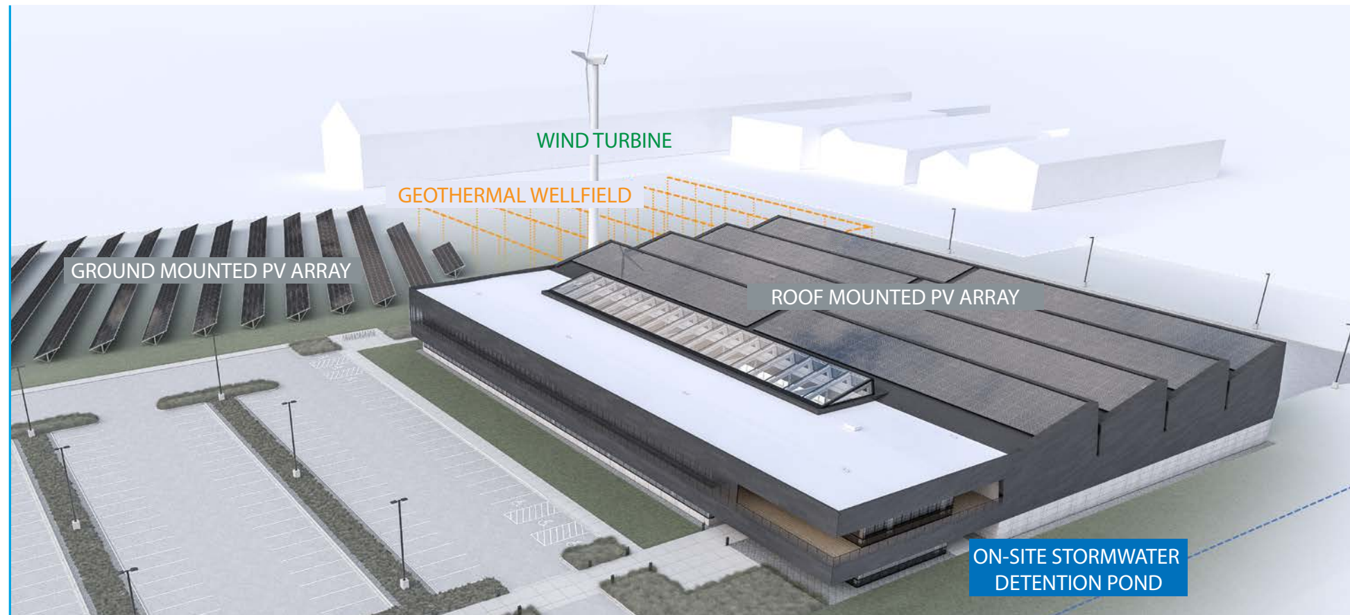
FIGURE 6. A zero energy light industrial manufacturing and commercial facility designed to achieve zero or better in several sustainability categories: energy, carbon, water, waste, materials, and value on an Erie County (New York) brownfield site
