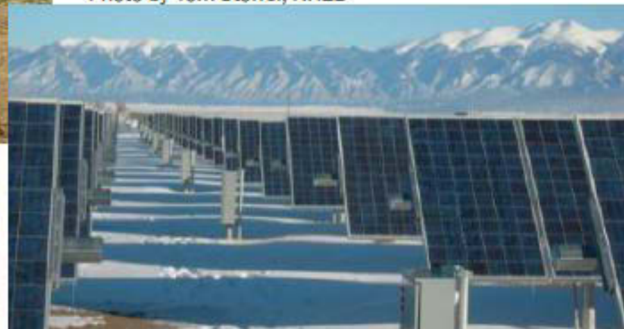
Alamosa PV System, Alamosa, Colorado Photo by Tom Stoffel, NREL
