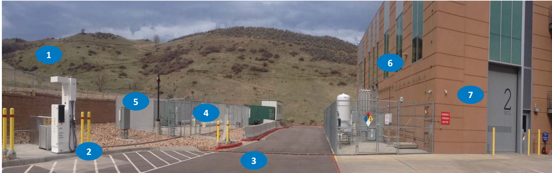
Energy Systems Integration Facility (ESIF)
