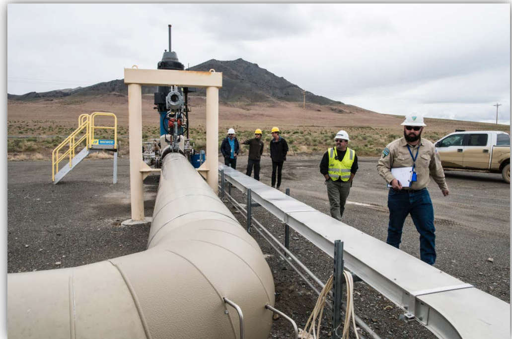
Blue Mountain Geothermal Power Plant, Humboldt County, NV Photo credit: Dennis Schroeder
