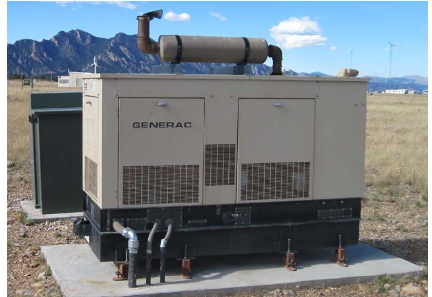
Source: NREL Pix 24490
