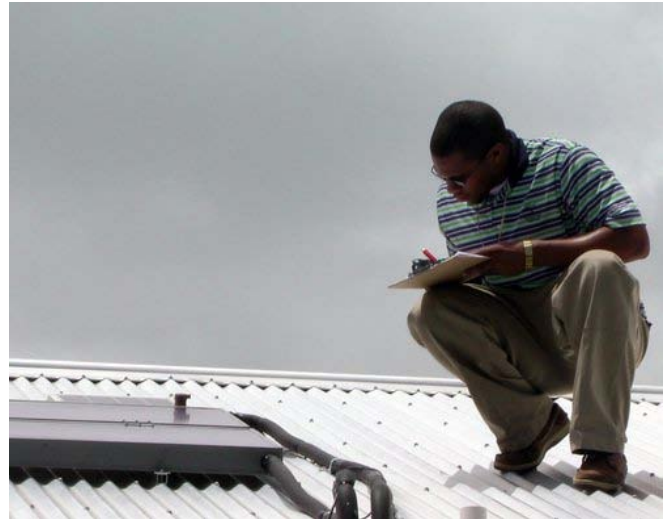
Figure 2. A Virgin Islands Energy Office intern inspecting a rooftop solar collector—St. Croix, U.S. PIX19339
