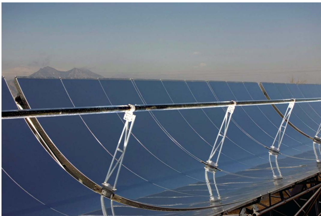
Figure 1. The black tube illuminated in center of this concentrating solar-thermal power parabolic trough collector is the receiver.
