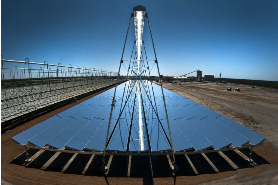
Figure 3. Fresnel concentrating solar power collectors comprise many thin, flat mirror strips that run parallel to the receiver. Each collector rotates on a single axis to keep the sun focused on the stationary receiver throughout the day.
