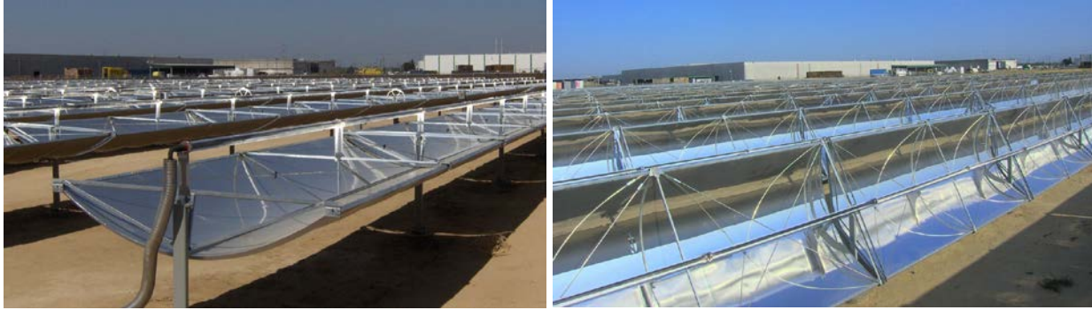
Figure 26. PTCs at the Frito Lay Modesto food processing plant 105
