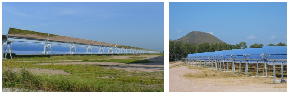
Figure 6. TSE1 site in Thailand where the Solarlite SL 4600s were being utilized for DSG 36
