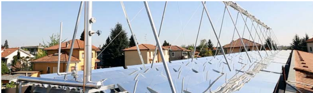
Figure 7. LF system installed on a roof 40
