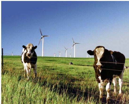
Wind farm co-located with a cattle operation.
