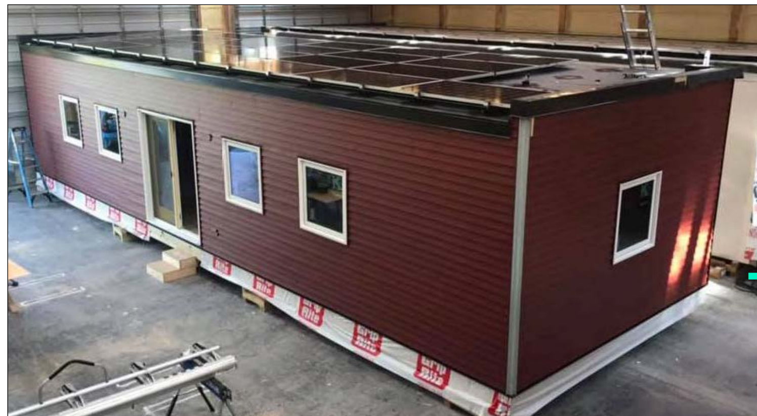
FIGURE 5 NZE modular units with factory-installed rooftop solar PV at the Solar Home Factory at Geneva, NY. Source: Solar Home Factory.
