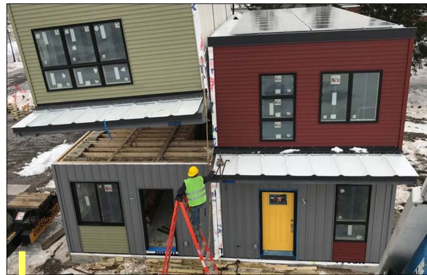
FIGURE 40 Solar Home Factory's volumetric modular units with factory-installed rooftop solar PV being set on-site. Source: Solar Home Factory.
