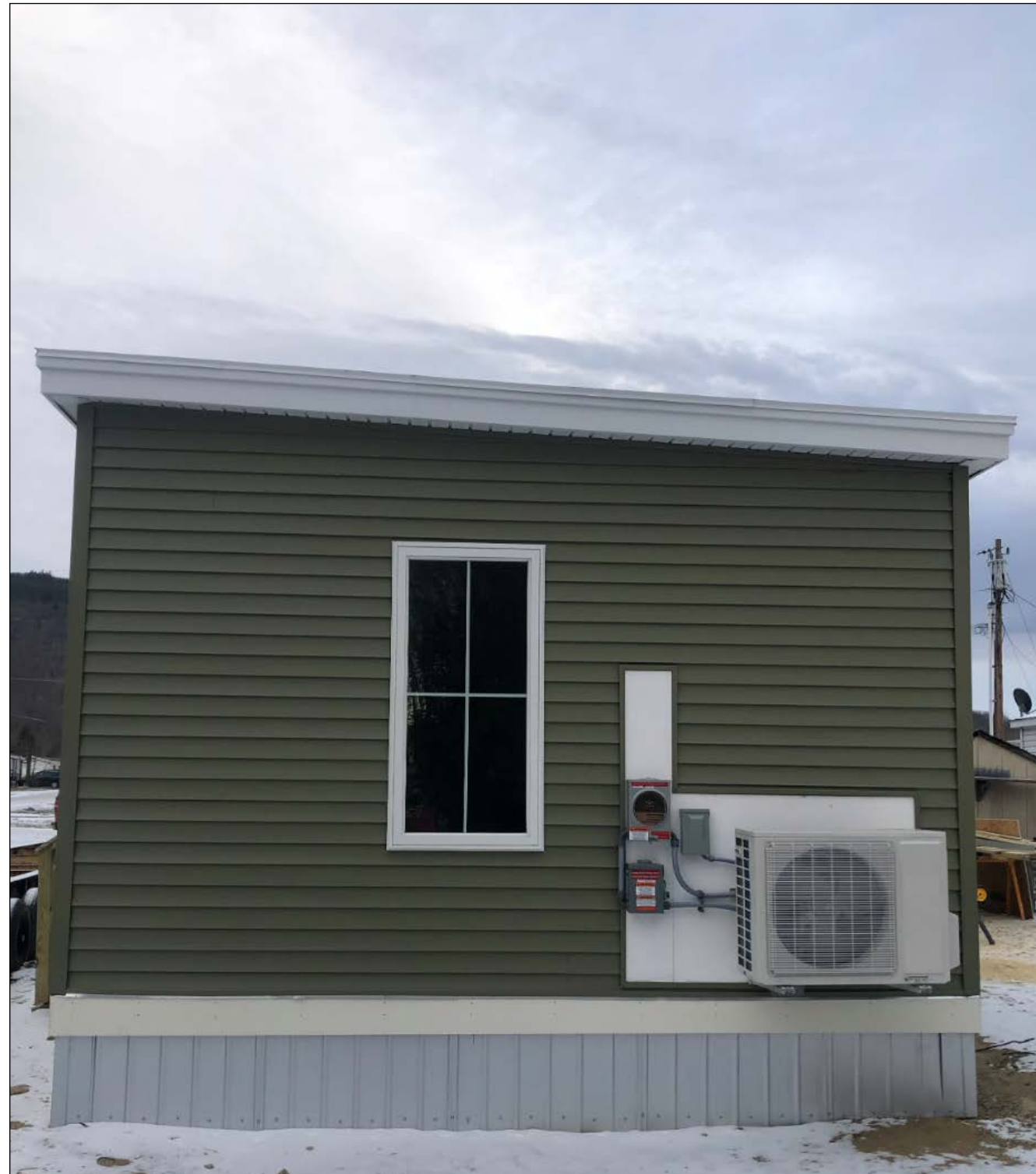
FIGURE 32 Photo documentation of VEIC's Energy Exchange Pod for zero-energy modular homes (partially implemented design option). Source: VEIC.
