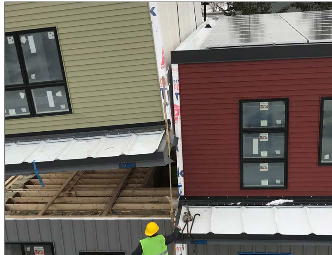
FIGURE 42 Solar Home Factory's dwellings are pre-assembled in the factory and shipped to the site, reducing on-site construction to civil, foundations, and exterior finish. Source: Solar Home Factory.
