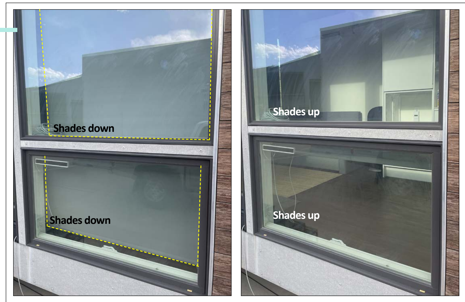
FIGURE 38 Dynamically controlled shading, triggered by DR events. Source: NREL.
