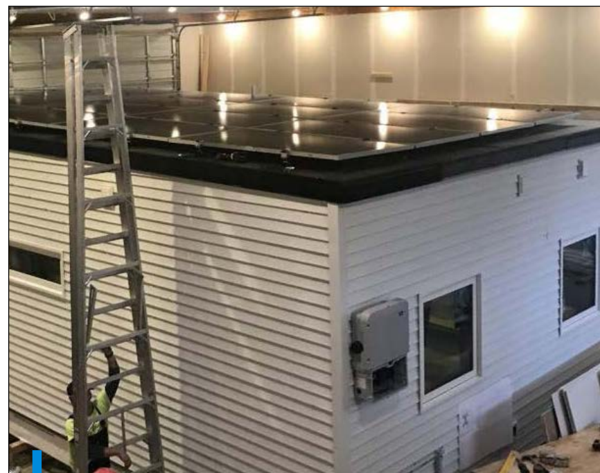
FIGURE 13 NZE modular housing unit, with rooftop solar PV, fully completed in the factory. Source: Solar Home Factory.
