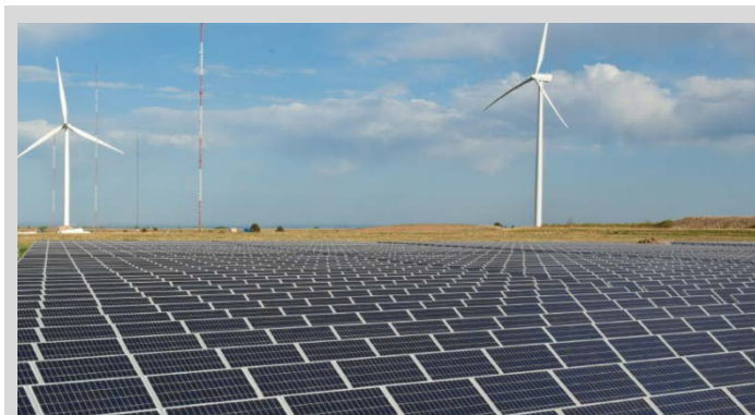
The FlexPower project will help accelerate the adoption of utility-scale variable wind and photovoltaic resources by demonstrating how hybrid power plants can provide essential reliability and resiliency services to the grid. Photo by Dennis Schroeder, NREL 20691
