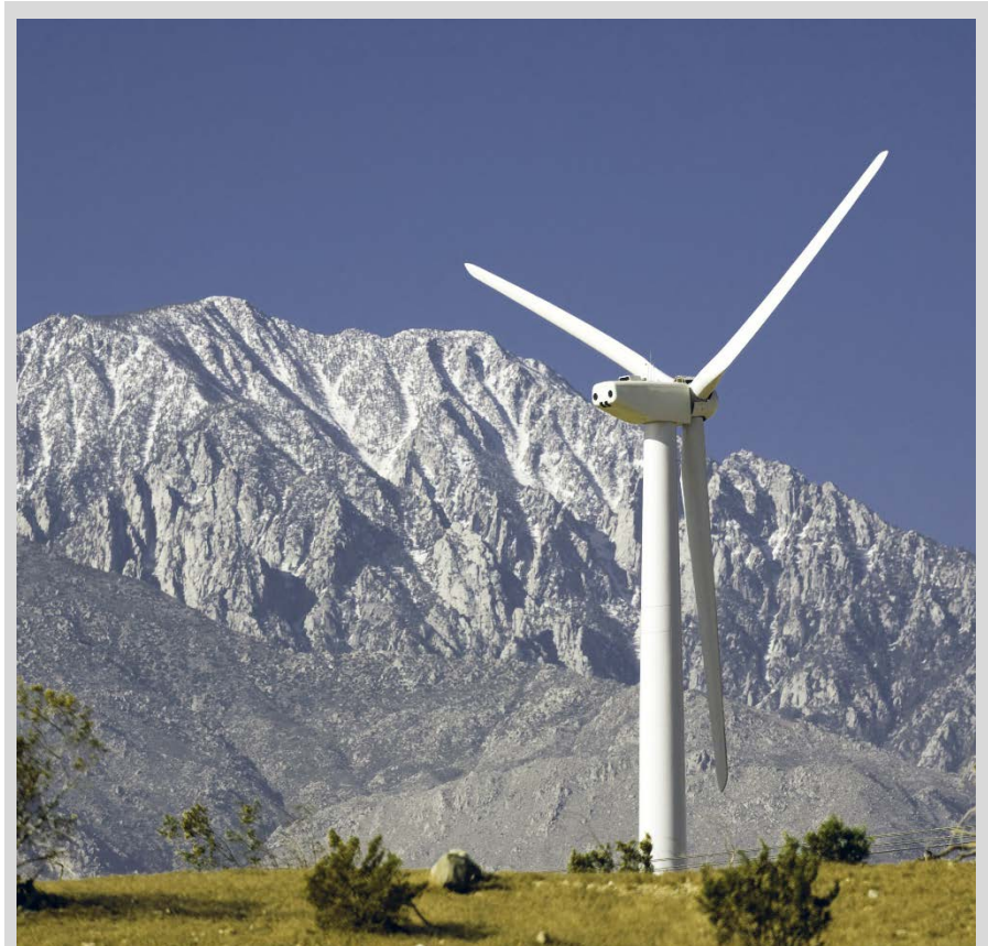
The ascent of stably stratified air over a mountain barrier can trigger the generation of mountain waves that can impact annual energy production at wind facilities. Photo from Iberdrola Renewables, NREL 16105
