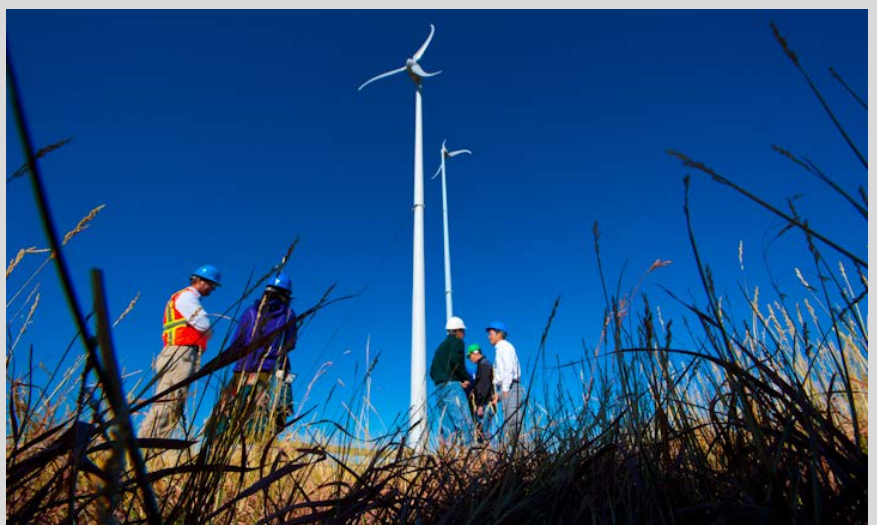
Minimizing material use and manufacturing cost while increasing annual energy production is important for the continued adoption of small wind turbines like the Southwest WincsdPower Skystream turbines shown here on NREL's Flatirons Campus. Photo by Dennis Schroeder, NREL 36248
