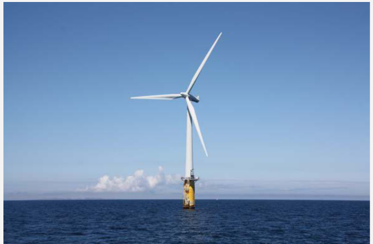
An NREL model predicts floating offshore wind could unlock new regions to offshore wind development, such as the Oregon coast. Photo by Senu Sirnivas, NREL 27606
