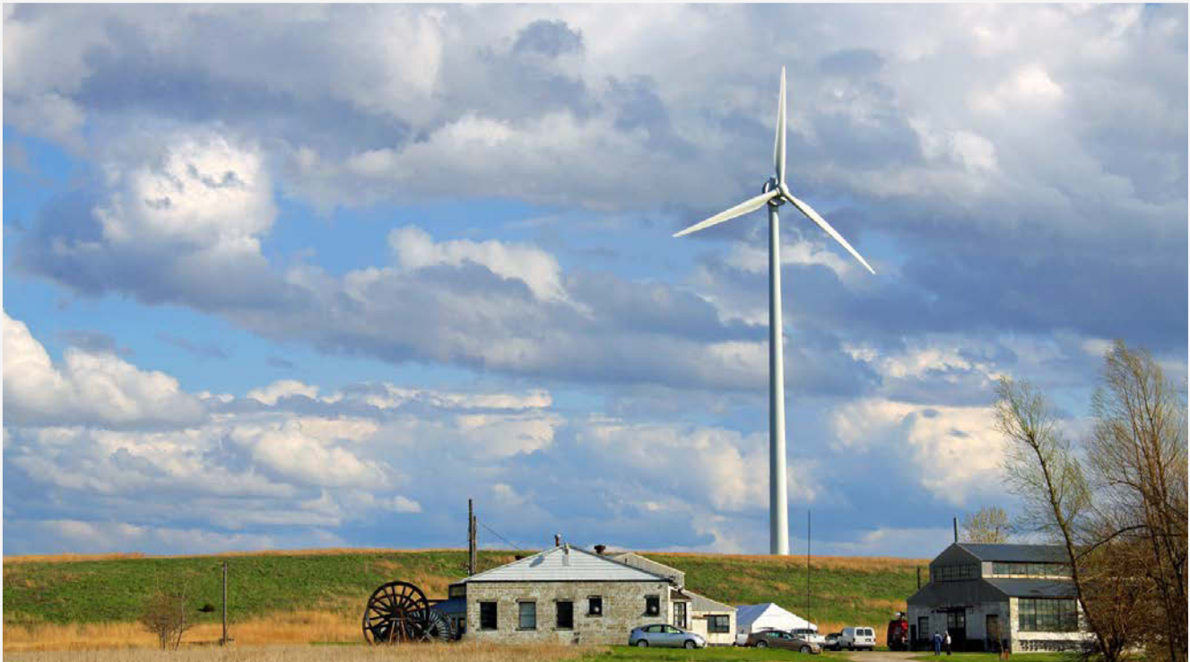
NREL's research on fault-tolerant control systems will determine how wind turbines could support isolated power systems. Photo by Rural Electric Convenience Cooperative
