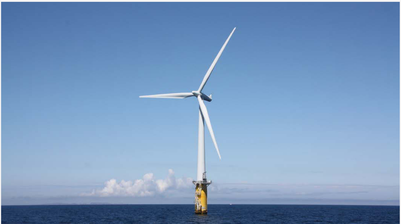
The WEIS project will develop an open-source, user-friendly toolset designed to enable offshore floating system engineers to design radically new systems at greatly reduced costs. Photo by Senu Srinivas, NREL
