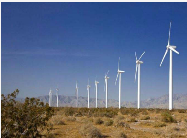
NREL collaborative research proves that wind power plants have the necessary controls in place to supply essential reliability services to the electric grid. Photo courtesy of Avangrid Renewables
