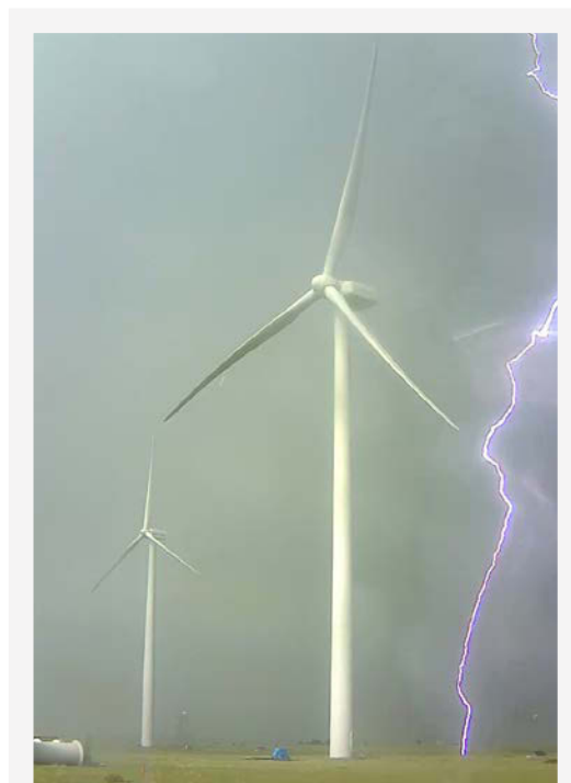
NREL researchers designed a 5-m blade tip section to protect thermally welded turbine blades from lightning strikes. Photo by Andrew Scholbrock, NREL 34113
