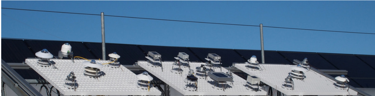
Figure 3-23. Test facility to quantify PV reference cell characteristics and compare them with other types of radiometers. Photo by PV Performance Labs
