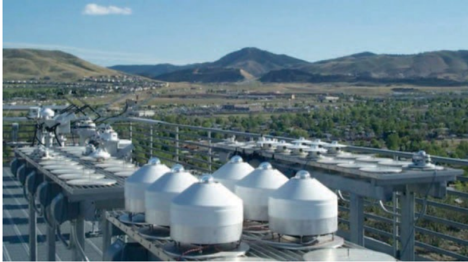
Figure 3-9. Kipp & Zonen model CM22 pyranometers installed in ventilated CV2 enclosures. Photo by NREL
