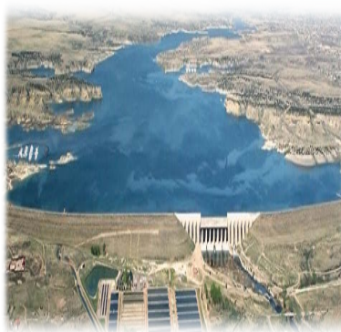
Figure 1. Southeastern Colorado Water Conservancy District – 7.5 MW Pueblo Dam Project. Photo courtesy of the CWCB
