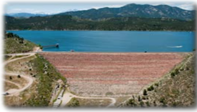
Figure 6. Northern Colorado Water Conservancy District – 1.3 MW Carter Lake Reservoir Project. Photo courtesy of CWRPDA
