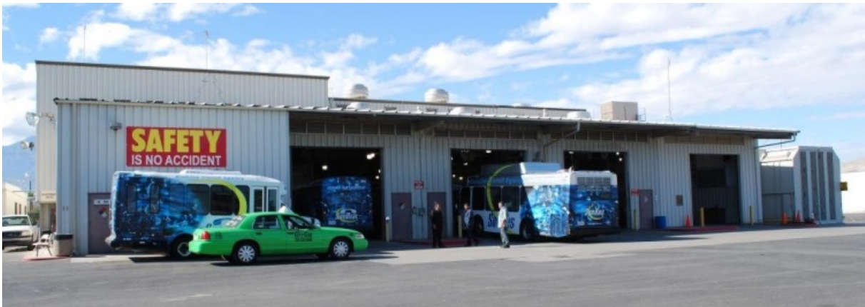
Figure 6. SunLine's maintenance facility
