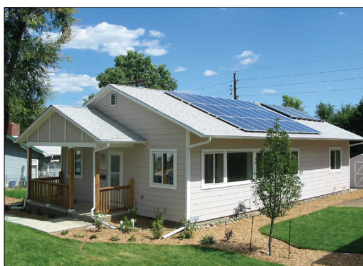
BEopt was used to find the most affordable combination of insulation, efficient equipment, and passive and active solar to reach the ZNE goal. The south-facing windows are well shaded by the roof overhang.
