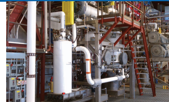
Photo by Dennis Schroeder, NREL/PIX 19528
