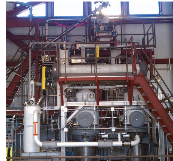
Photo by Dennis Schroeder, NREL/PIX 19527
