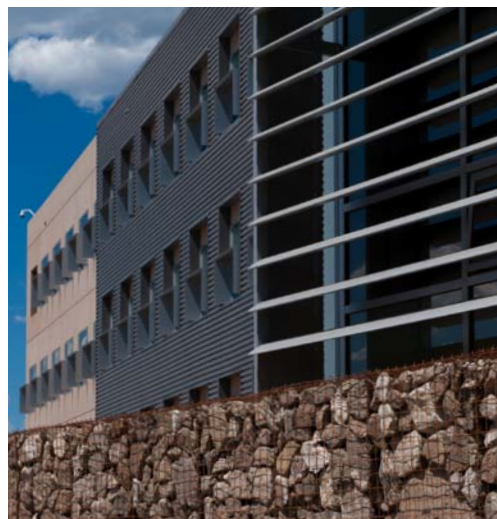
Gabion walls. Photo from Frank Ooms Photography
