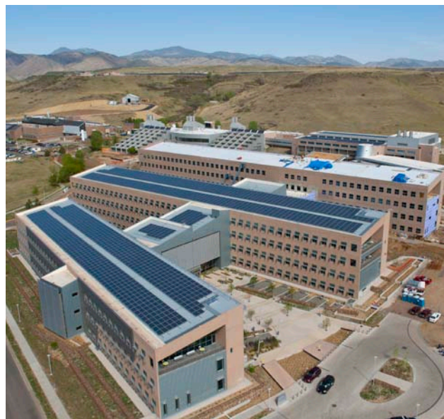
The RSF includes 450kW of roof-mounted PV panels. Photo by Dennis Schroeder, NREL/PIX19089
