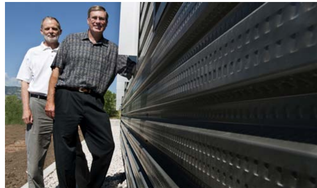
NREL researchers next to their award-winning transpired solar collector on the RSF's south wing. Photo by Dennis Schroeder, NREL/PIX 17659
