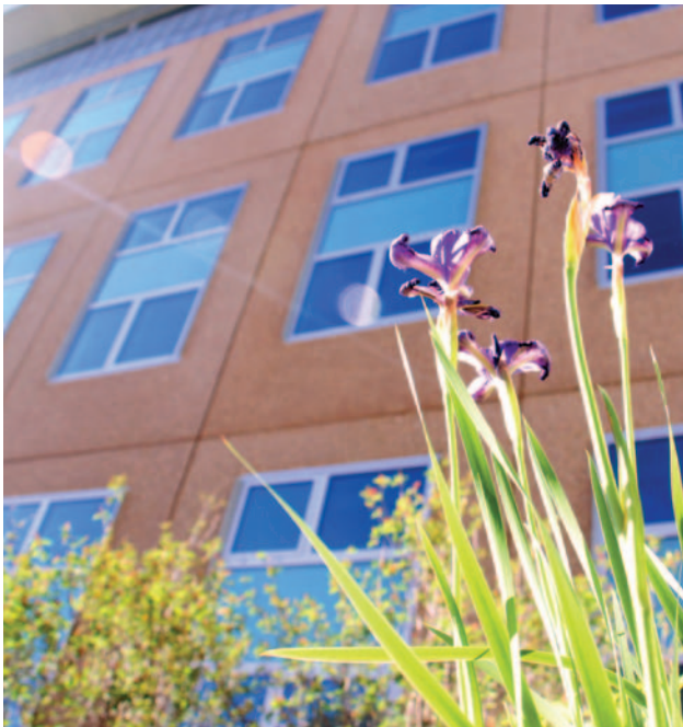
The RSF serves as a blueprint for achieving ultra-energy efficiency and net-zero energy performance. Photo by Heather Lammers, NREL/PIX 17515
