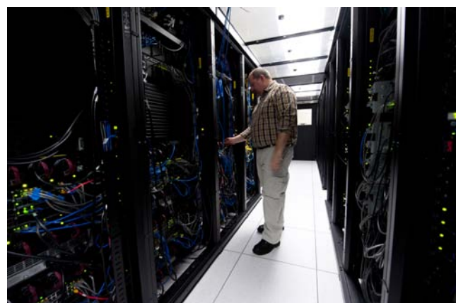
The RSF data center features an extremely low power usage effectiveness ratio of 1.13. Photo by Dennis Schroeder, NREL/PIX 18780
