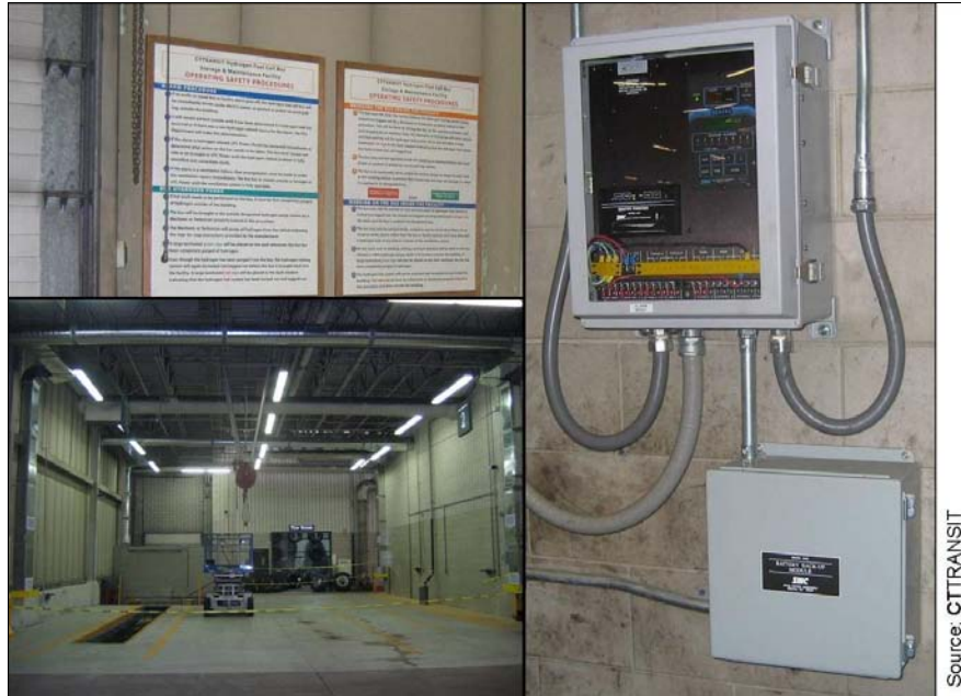
Figure D-1. CTTTRANSIT fuel cell bus maintenance bay (lower left), operating procedures (upper left), and alarm control system (right)
