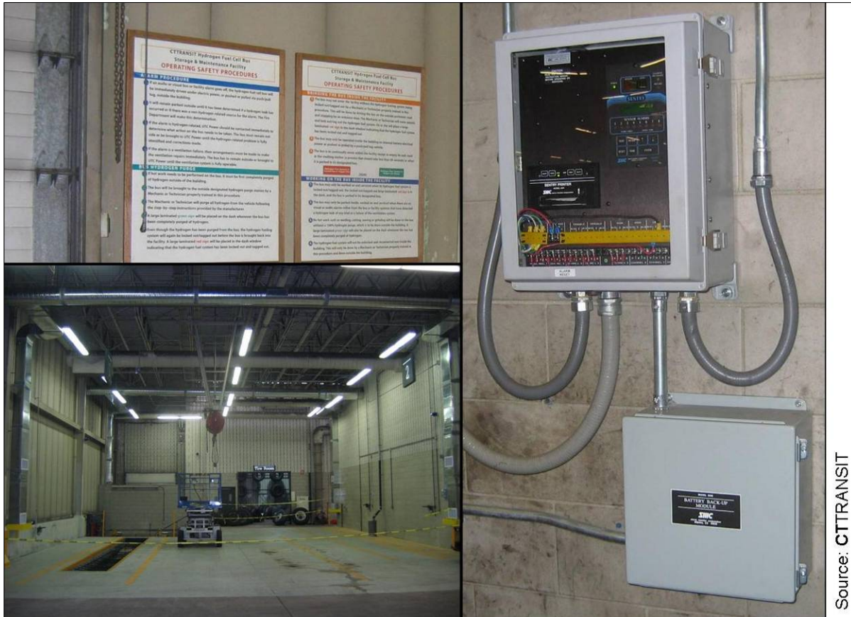
Figure 6. CTTRANSIT fuel cell bus maintenance bay (lower left), operating procedures (upper left), and alarm control system (right)
