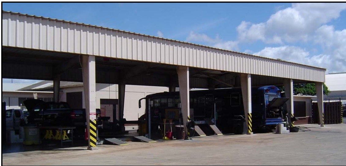
Figure 10. The open-air maintenance facility at Hickam
