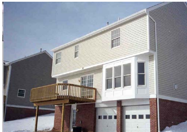
Figure 7. Home used for CFD thermal case study (Cases 8 to 10), built by Heartland Homes in Pittsburgh, Pennsylvania. Courtesy of the Building America Program [17].
