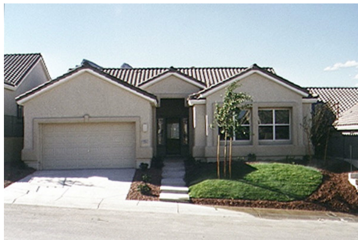
Figure 3. Home used for isothermal CFD case study (Cases 1-7), built by Pulte Homes in Las Vegas, Nevada. Courtesy of the Building America Program [17].
