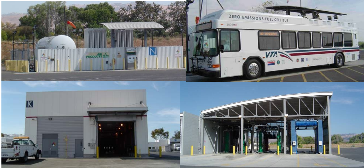
Figure ES-1. Compressed hydrogen dispensing station, fuel cell bus, bus wash, and maintenance facility
