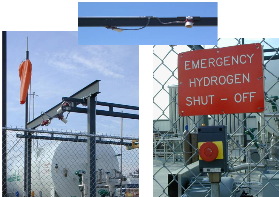
Figure 6. Flame sensors (left and top) and emergency shut-off (right) at the hydrogen dispensing facility
